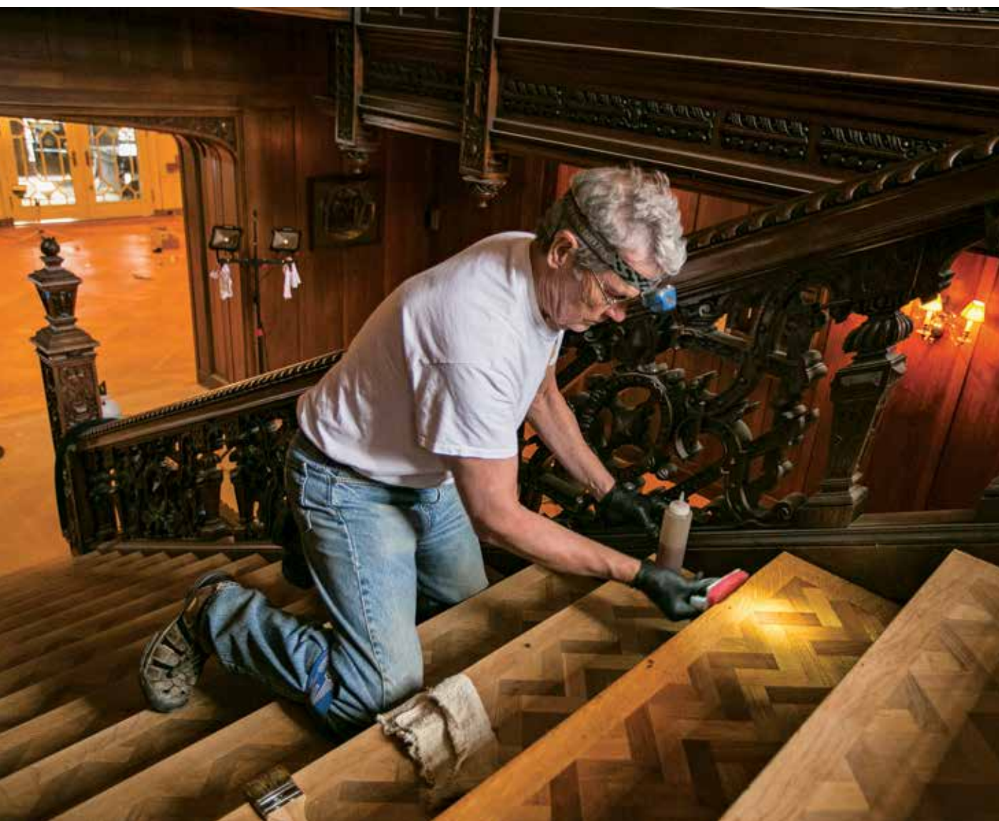
Fair Lane's white oak floors were laid in a herringbone pattern, including staircases and closets. Photo by John F. Martin.
